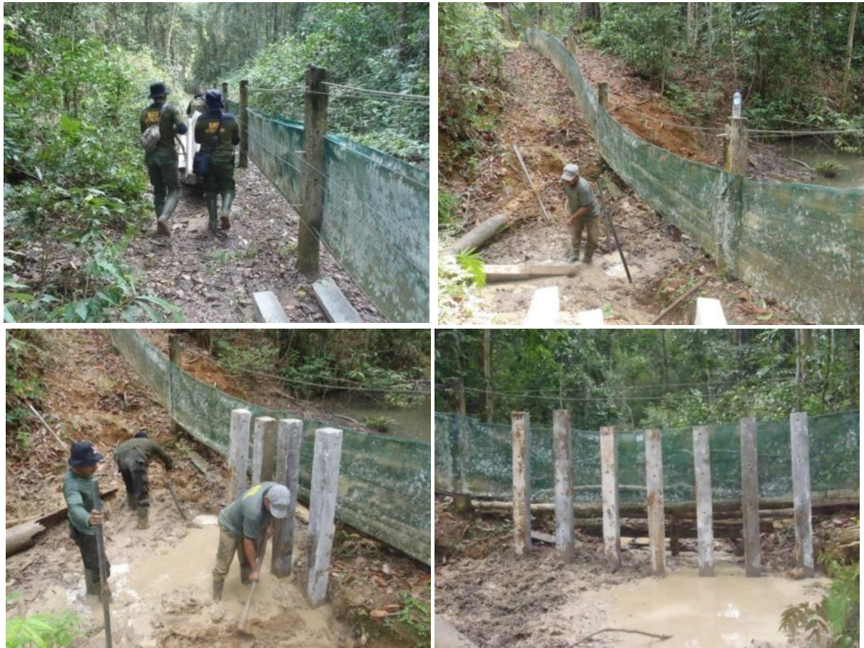
Figure : SRS's staff repaired the fences facility in the swamp area (between 1-5 fences and 4-5 fences), before we used tree and now changed with concrete pole.
