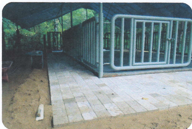
cage floor and plug cement paving blocks
