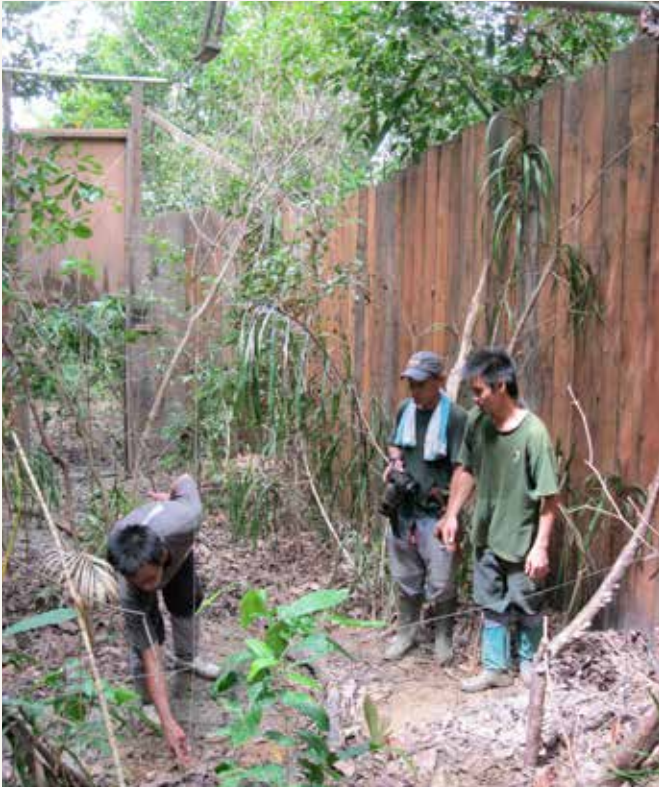
Rhino trap designed for the possibility of two rhinos traveling together : a small paddock with hardwood fence and door at each end, built on a rhino trail. When a large animal enters the trap, it will push a central arrangement of barely-visible, fine plastic-coated wires, that pull a steel plate downwards and simultaneously releases ironwood pegs, cables and both doors within 1 second.
