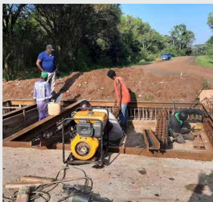
An elephant grid under construction.
