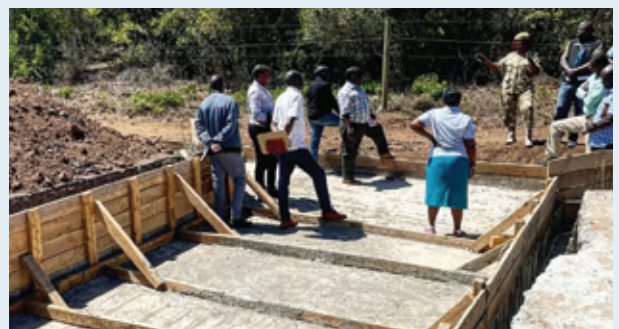
Elephant grid under construction in Upper Imenti
