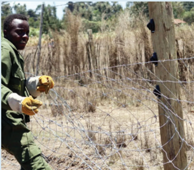
Fence attendant straining a tight-lock wire mesh
