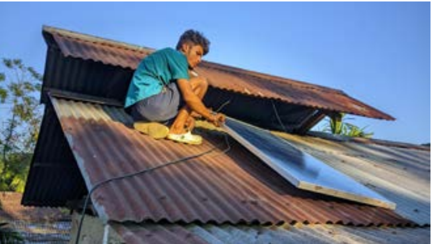
Installation of solar panel to energise solar fence in a HEC-affected area
