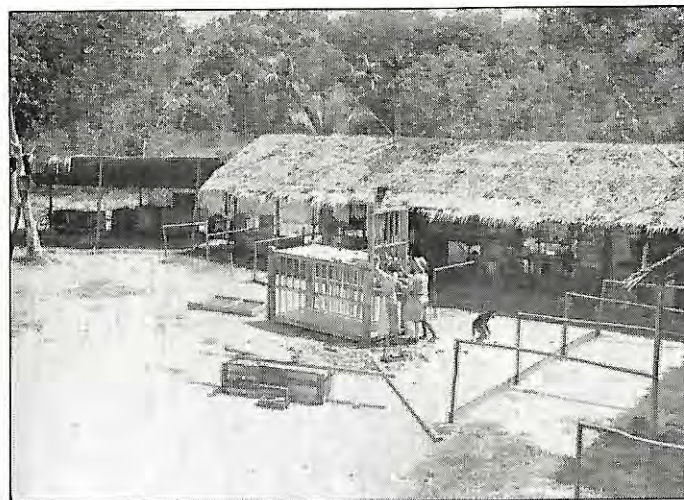
A permanent camp has been set up in a cleared space in the jungle. The men are at work building a rhinoceros cage.
