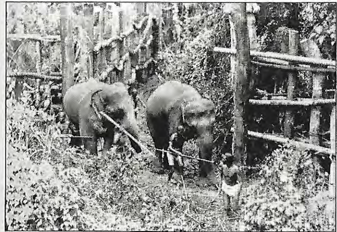
One elephant can do the work of twenty men in hauling the great logs which make this fence in the jungle of Ceylon.
