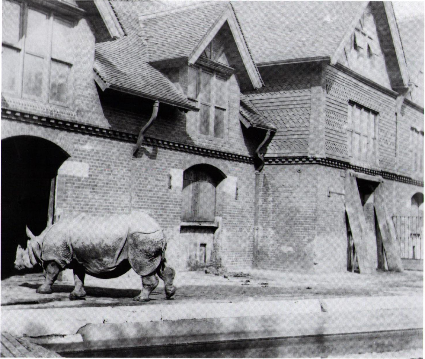
Jim entering his stall, circa 1900. Note the timber buttresses, a relic of Jumbo's residence and the recessed drainpipes, to prevent damage from the animals.
