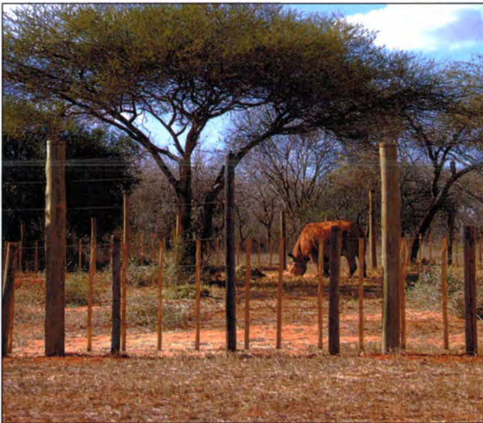
The fencing of the natural enclosure was visually highlighted using added poles shorter than the main poles plus adhesive tapes. (dh)
