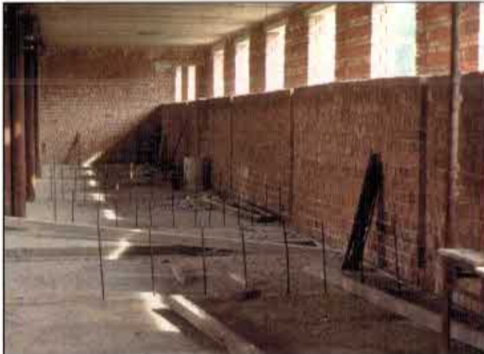
The new rhino house in the construction period prior 1990 (pch)
