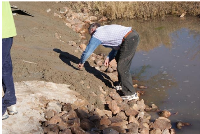
Figure 3: Pushing the cement in between the rocks
