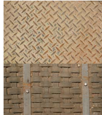
Steel “fish plate” (top) and woven rubber matting (bottom) give good footing in a transport crate.
