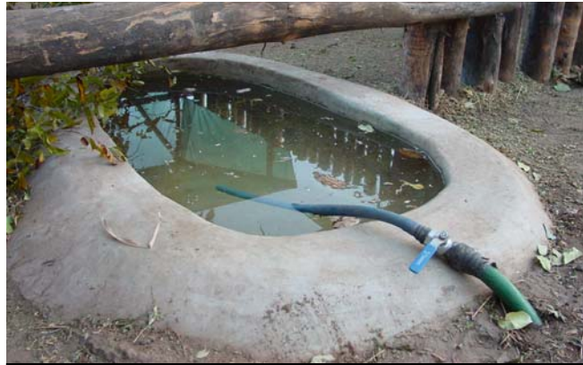
Water trough with concrete skirt, hosepipe to fill, emptied with a bucket (looking from outside in)
