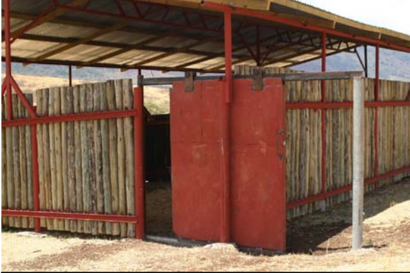
Boma door with beam at top and bottom. Boma walls supported by vertical poles and horizontal channel.
