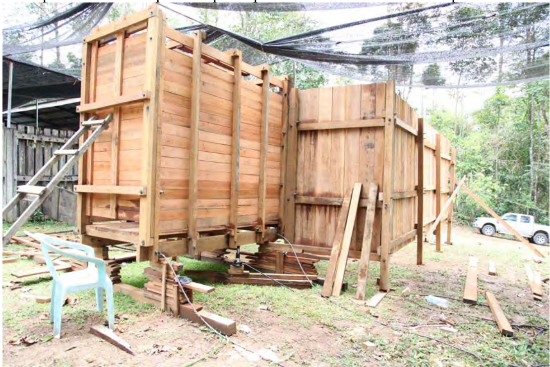
Rear quarter view of trap with boma attached. The lower part of the posts will be dug into the ground.
