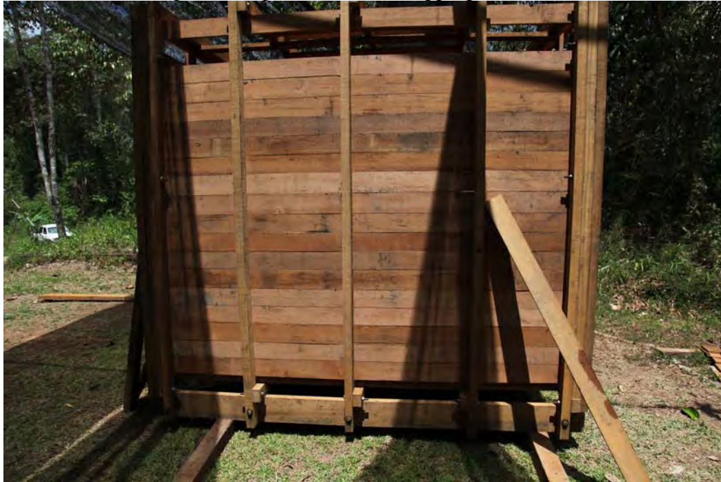
Side view. 7,5 feet long – 8 ft high. The frame in both end consists of three 2x4 in posts. The three posts in the middle are 2x3 in. The bottom post is 2x6.
