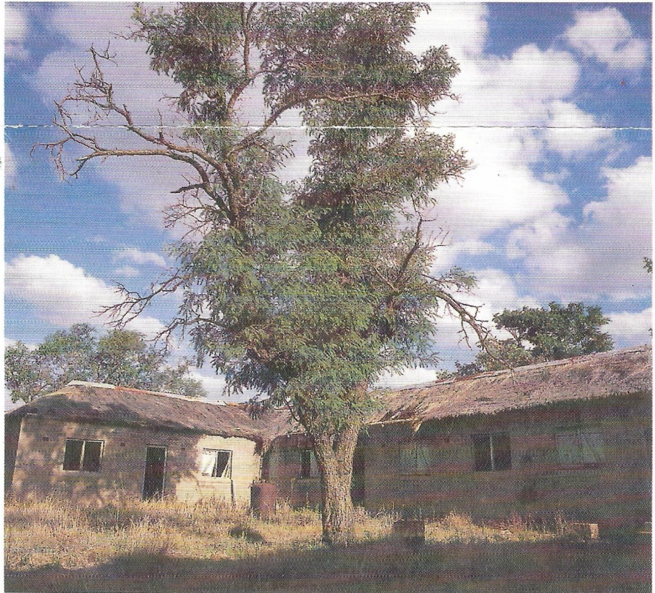
Girls' dormitory prior to renovation, November 1996
