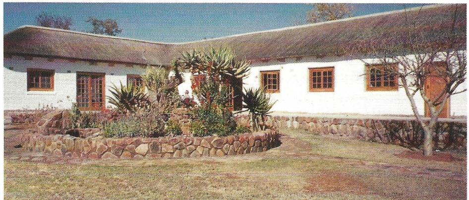
Girls' dormitory after renovations & restoration work, August 1998
