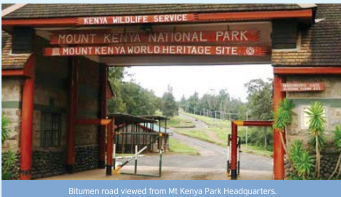
Bitumen road viewed from Mt Kenya Park Headquarters.
