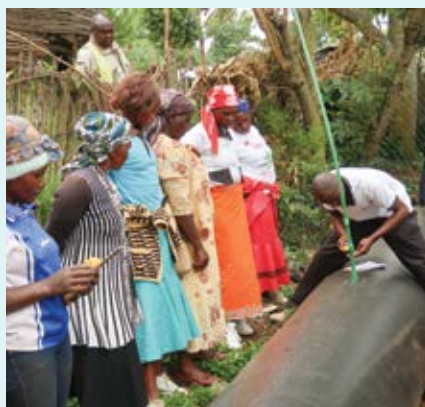
Biogas digester installation.
