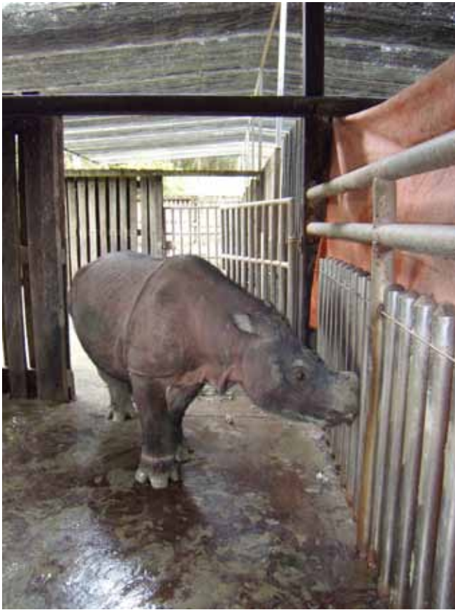
Interior of the old rhino night stall at Tabin after renovation
