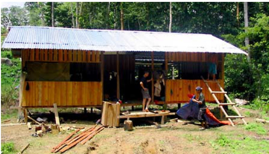
Constructing a new base camp. Photo Marc D Bowden
