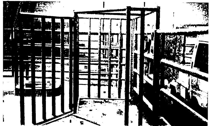
A free-stall chute that is incorporated into an enclosure can be particularly effective for relatively non-invasive procedures. Note how the angled entry and safety pipes allow a veterinarian or researcher access to the rear of the animal without the possibility of the animal's backing straight out. (Photo: Fossil Kin Wildlife Center)
