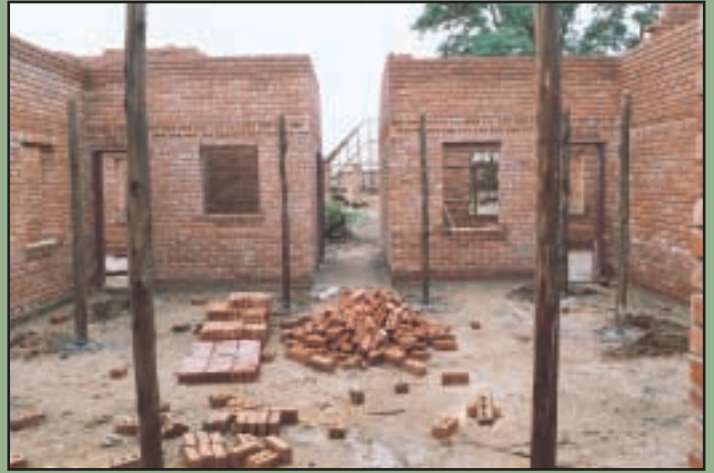
Looking into the courtyard of the office building
