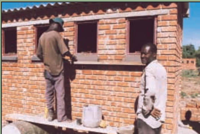
Forming concrete window sills
