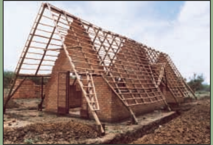
Dual bungalow accommodation building
