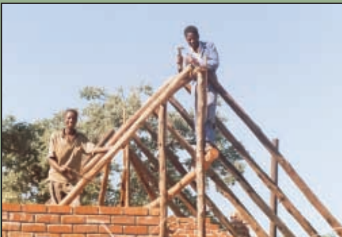
The roofing carpenters
