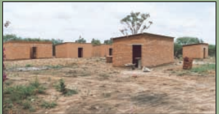
The staff accommodation blocks
