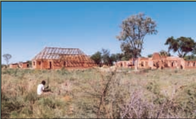
Looking across the site
