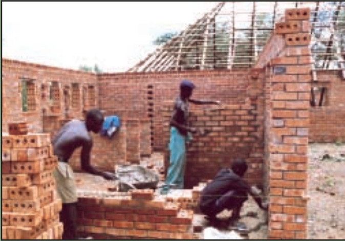
Brickwork for washroom / toilet block
